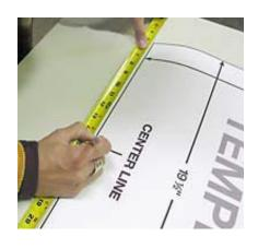
8) On this line, measure and mark the center point of the door from side-to-side.
