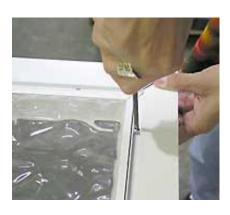
6) Once the pins are removed, carefully remove the door. Place the door on sawhorses, making sure the door is protected from scratching.
