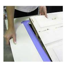
16) Set the block insert on the sawhorses with the side with the removed frame facing up. Place a 1/4" bead of caulk around the perimeter of the block insert frame approximately 1/2" from the edge. Leave a 1" gap in
